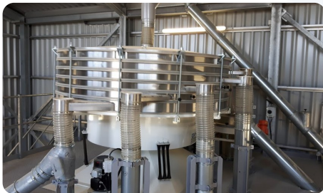
Tumbler screening in an industrial-sand plant
